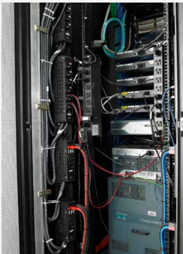
NetSure RDB H3 Deployed in a Knürr Rack
